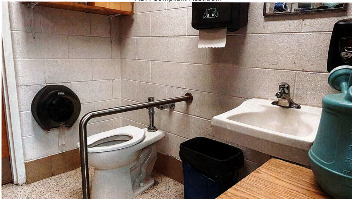
ADA Compliant Restroom
