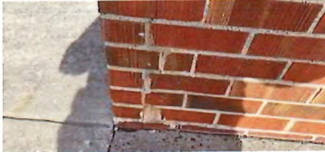
Photo 4: Cracked bricks
