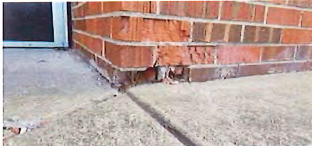
Photo 5: Missing/cracked bricks/spalling
