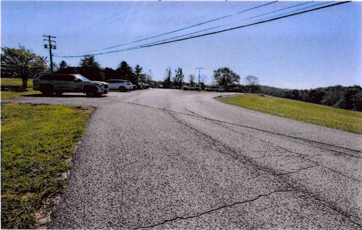
Parking Lot and Bus Loop
