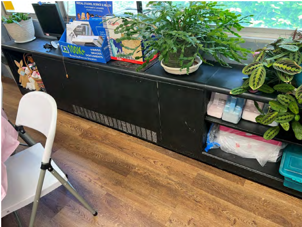
Old heating unit and bookshelves in classroom. Units no longer used.
