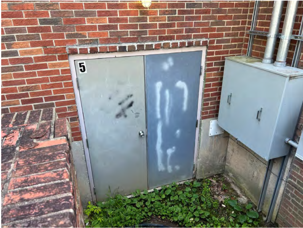
The door and landing are basement level. Sign a vegetation and water infiltration as a sump pump is located in the catch basin drain.
