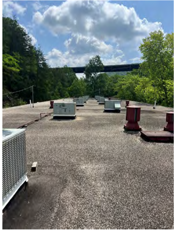
Roof area with existing rooftop mechanical units that are reaching life expectancy.
