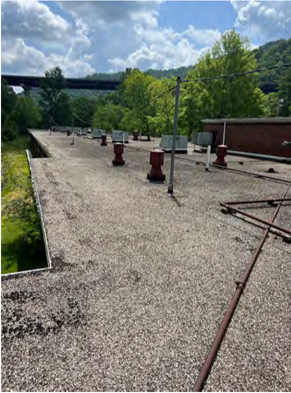
Roof area with existing rooftop mechanical units that are reaching life expectancy.
