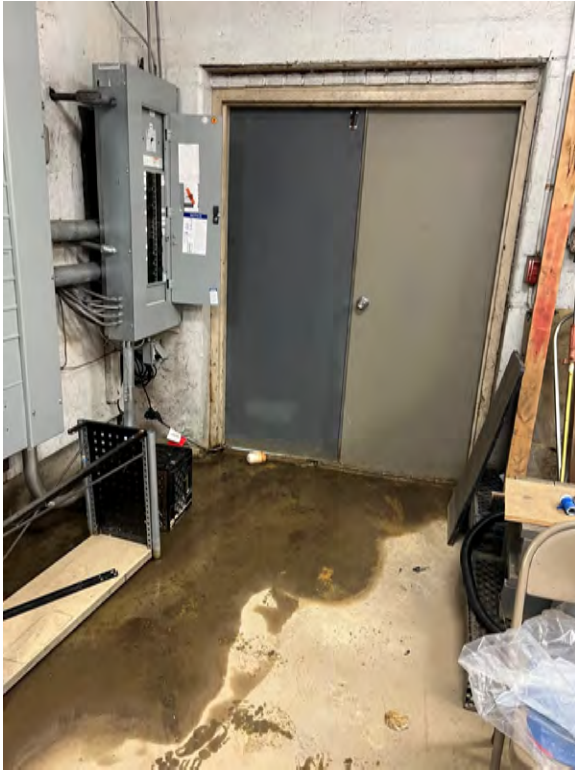
Basement with visible signs of water at the exterior door and base of stair from interior entrance.
