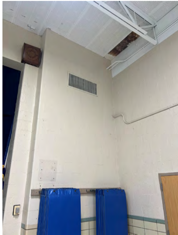
Roof leak in Foor storage area (left) and roof leak in multi-purpose room (right).
