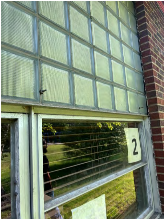
Glass block over existing windows showing through bolts and broke block
