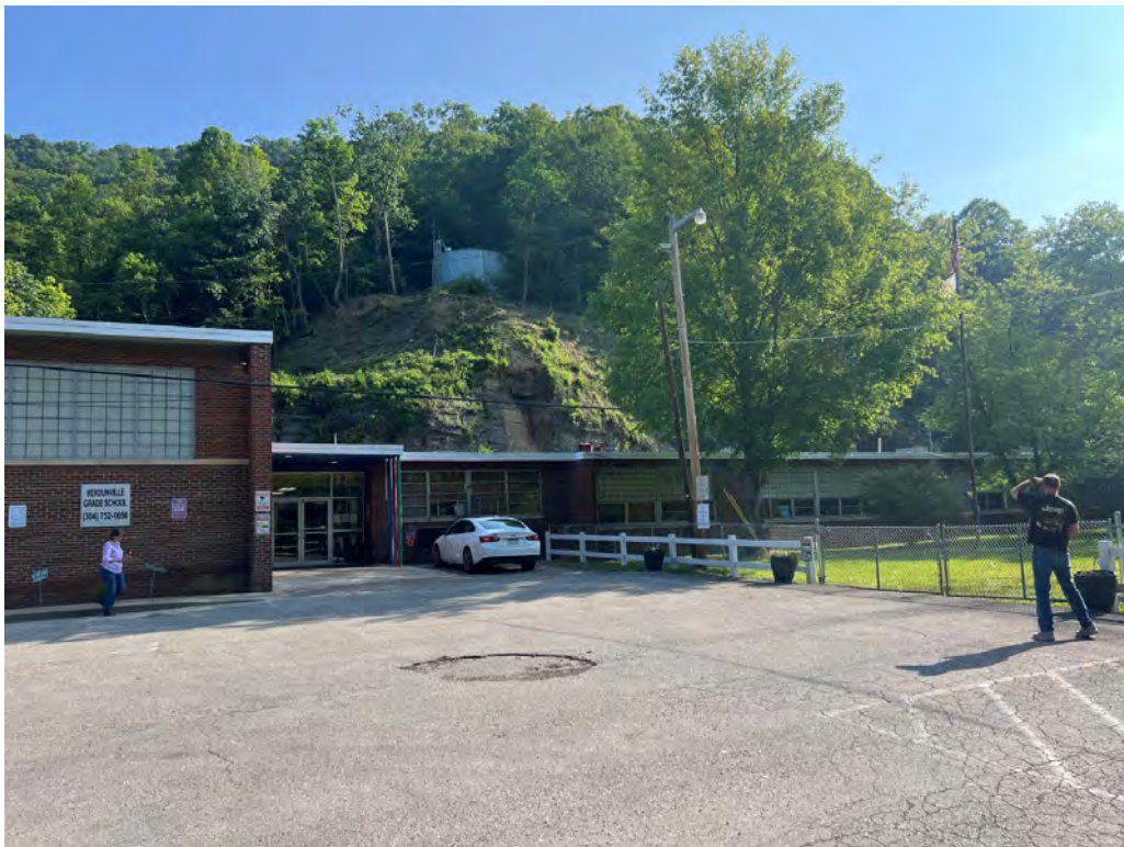
Front of the building with the main school entrance.
