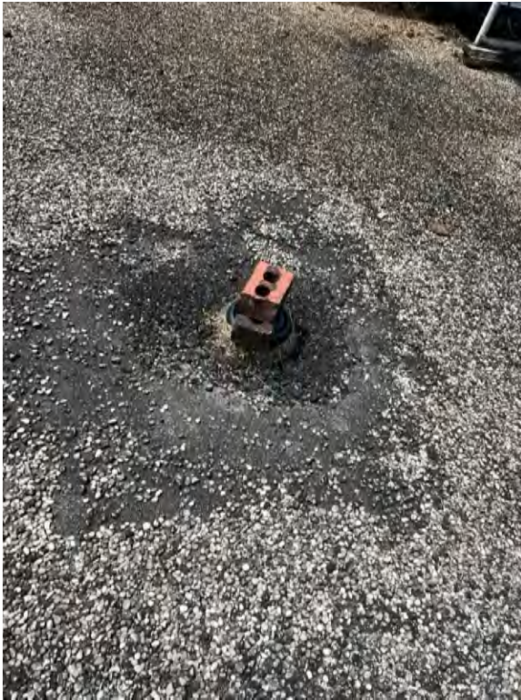
Roof drains with bricks on top to hold down the cover and vegetation growing around them.
