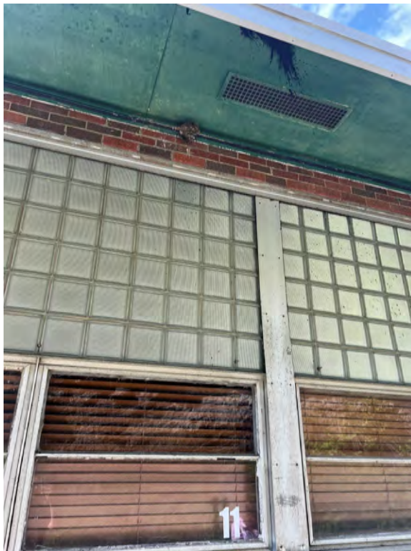
Overhang of the roof with a small, vented soffit.
