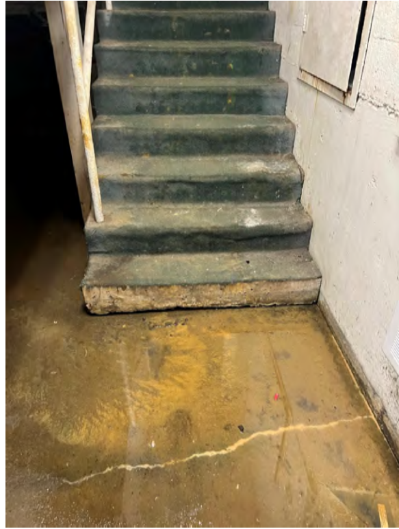
Basement with visible signs of water at the exterior door and base of stair from interior entrance.
