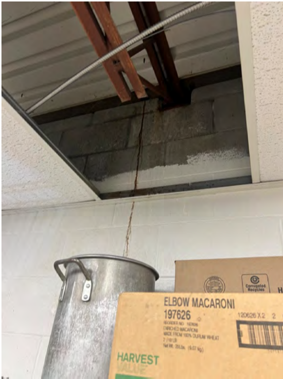
Roof leak in Foor storage area (left) and roof leak in multi-purpose room (right).
