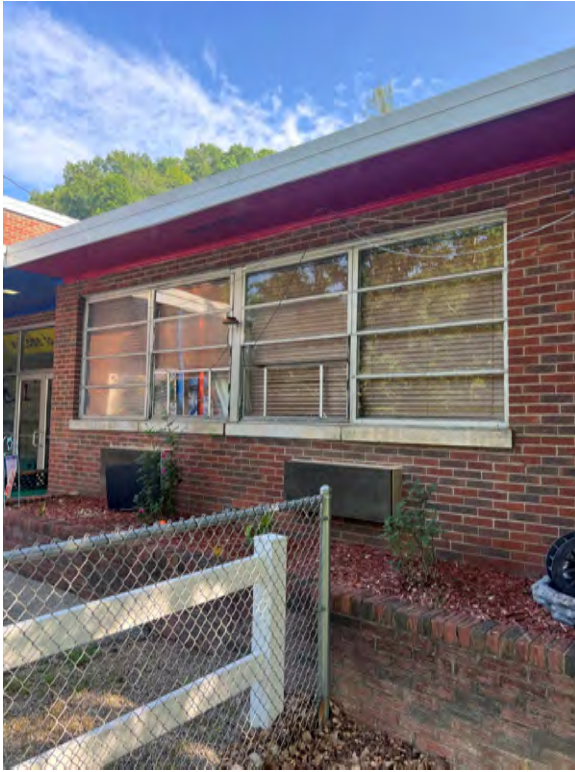
Original aluminum windows at General Office and typical classroom.
