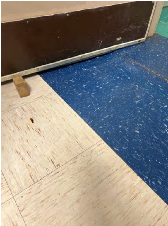
Sunken floor at the transition between the food storage and the stage. Masonry separation at the addition, not properly connected/sealed.
