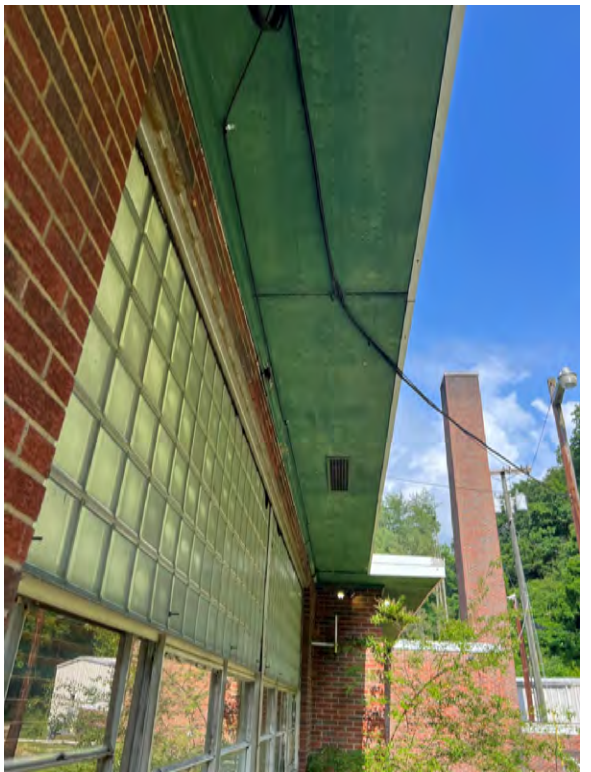
Overhang of the roof with a small, vented soffit.
