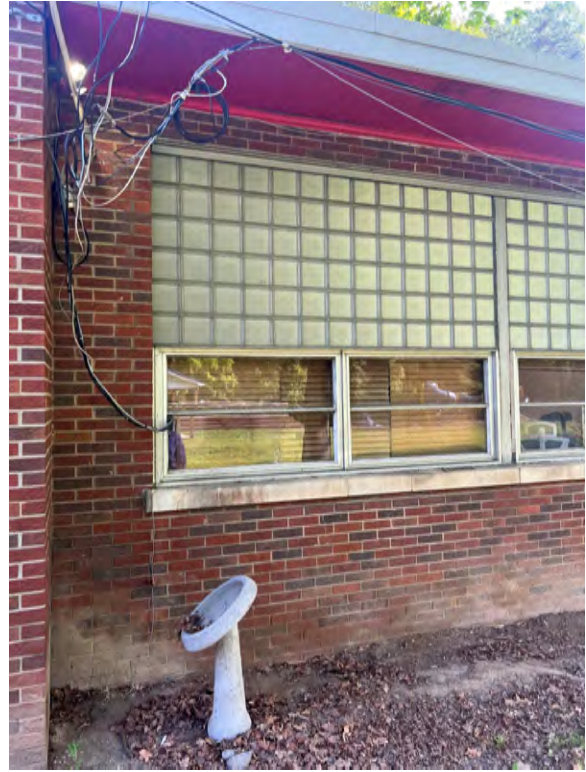
Original aluminum windows at General Office and typical classroom.
