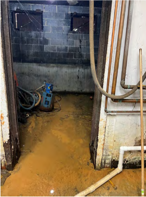
Standing water near old coal furnace area rusted door frame. Soap suds bubbling from drain from washer above in elevated janitorial space.
