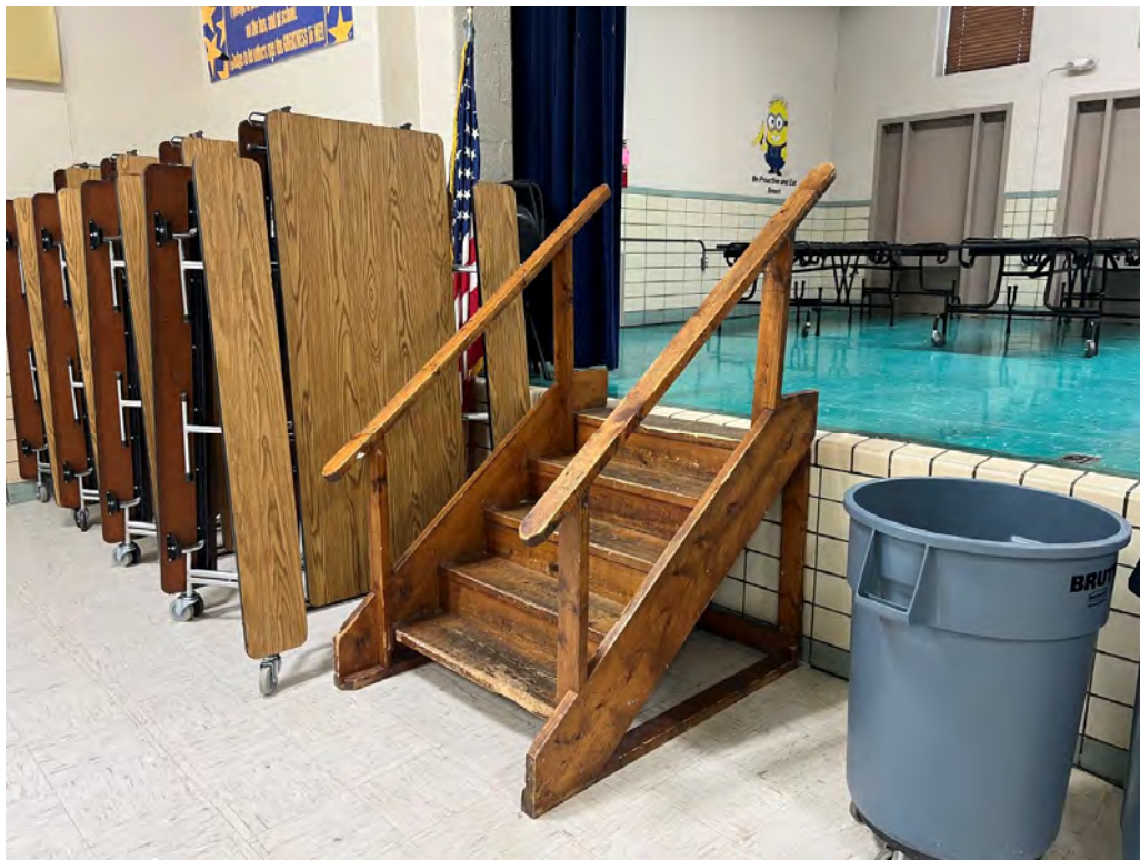
Wood stairs to the elevated stage area.
