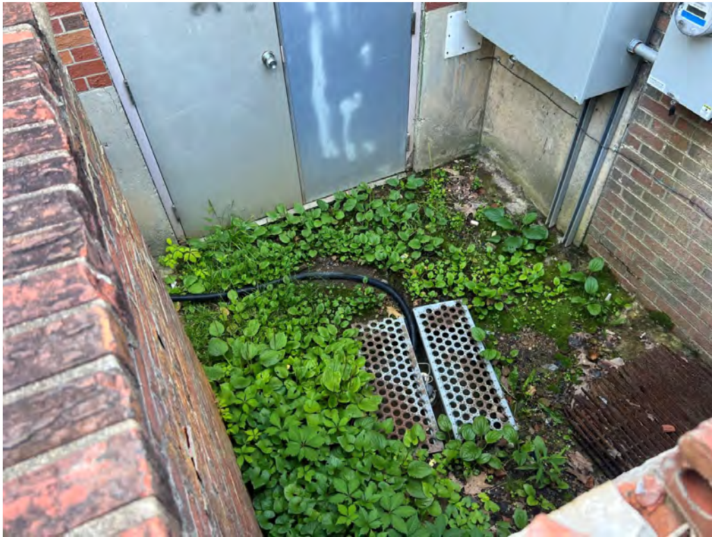
The door and landing are basement level. Sign a vegetation and water infiltration as a sump pump is located in the catch basin drain.
