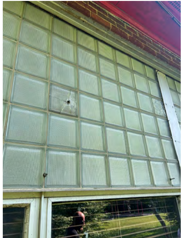
Glass block over existing windows showing through bolts and broke block
