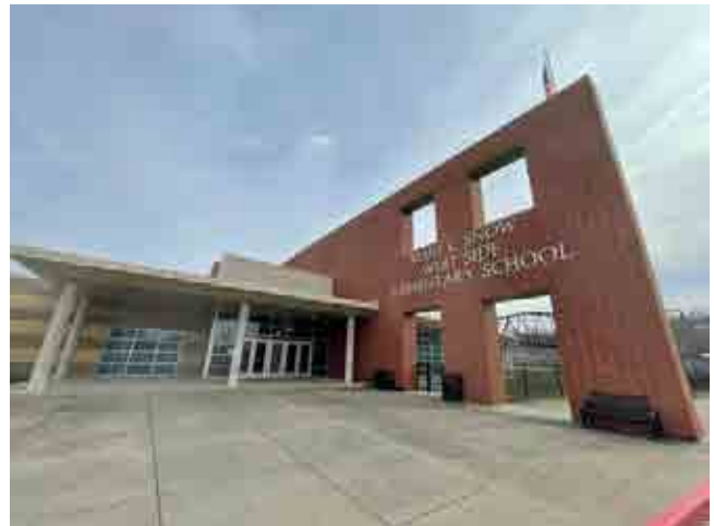
Mary C. Snow West Side Elementary School
