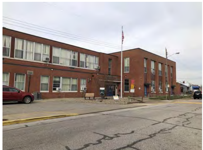
Bridgeview Elementary School
